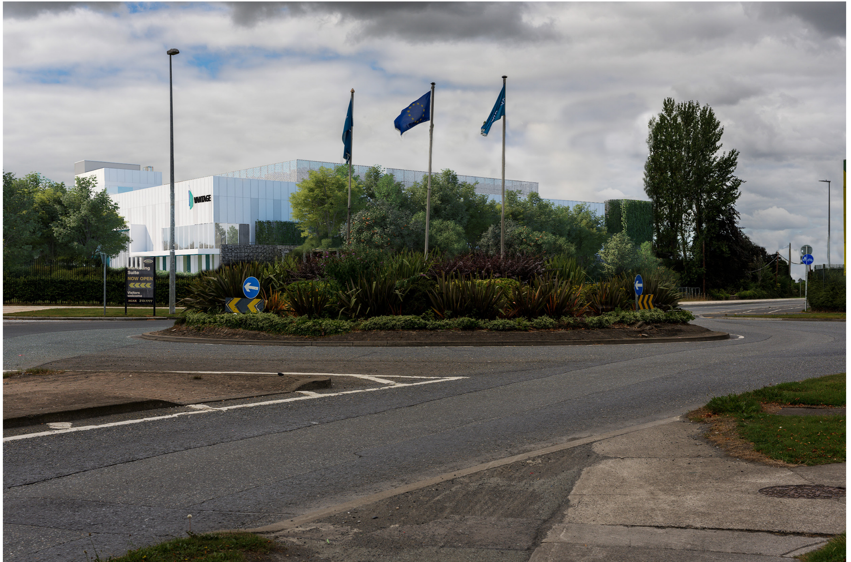
Viewpoint 7: Photomontage of Year 5 view from R134 New Nangor Road at the entrance to Profile Park | Viewing distance at A3: 542mm | Horizontal field of view: 39.6° | Direction of view: 252° Camera: Sony ILCE-1 | Lens: Sony 50mm | Camera height: 1.5m AGL | Date taken: 25 August 2022 | Aperture: f/8 | ISO speed: 100 | Shutter: 1/320 sec
