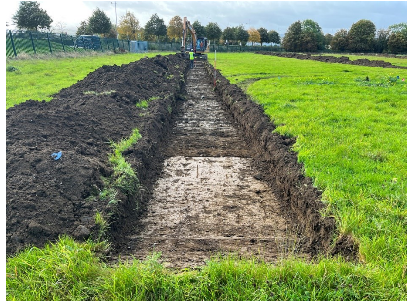
Plate 6: Trench 6 looking southeast.
