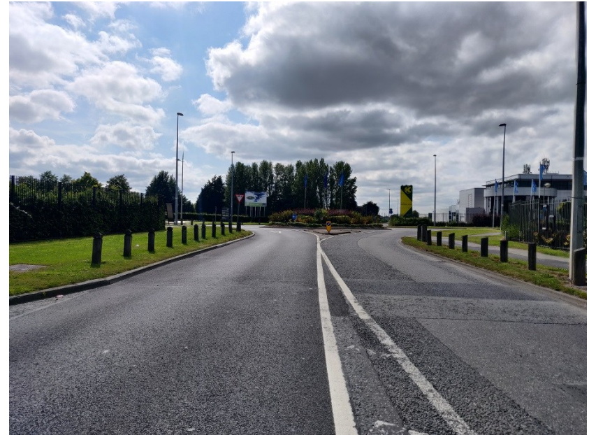
Plate 6: Roundabout at site entrance, looking west
