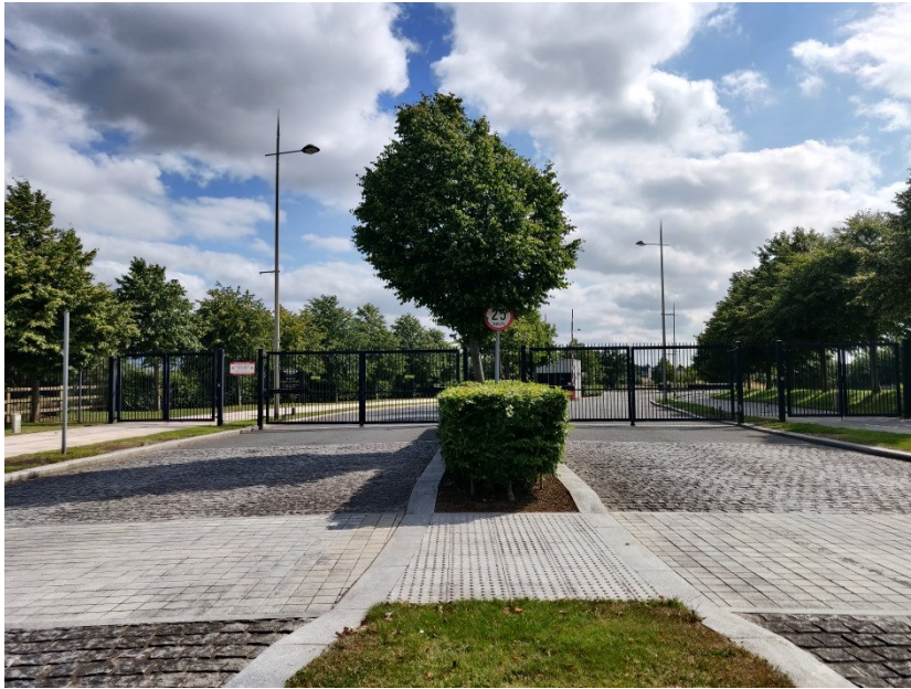
Plate 9: Site entrance, looking south
